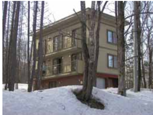
Figure 1. Appearance of CS treatment house
